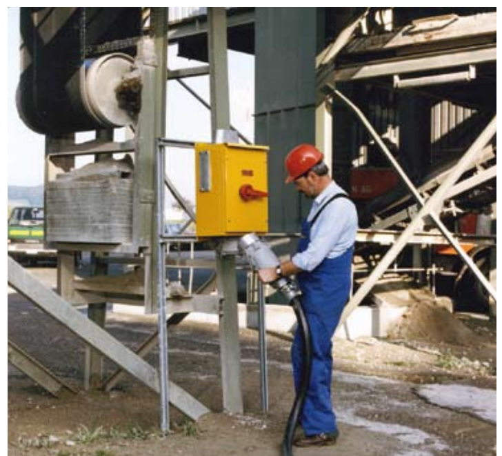
Gravel works: Switzerland
